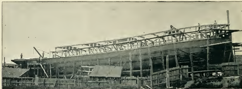
STEEL PROPELLER, 180 ft. by 40 ft., 15 ft. Hold.
